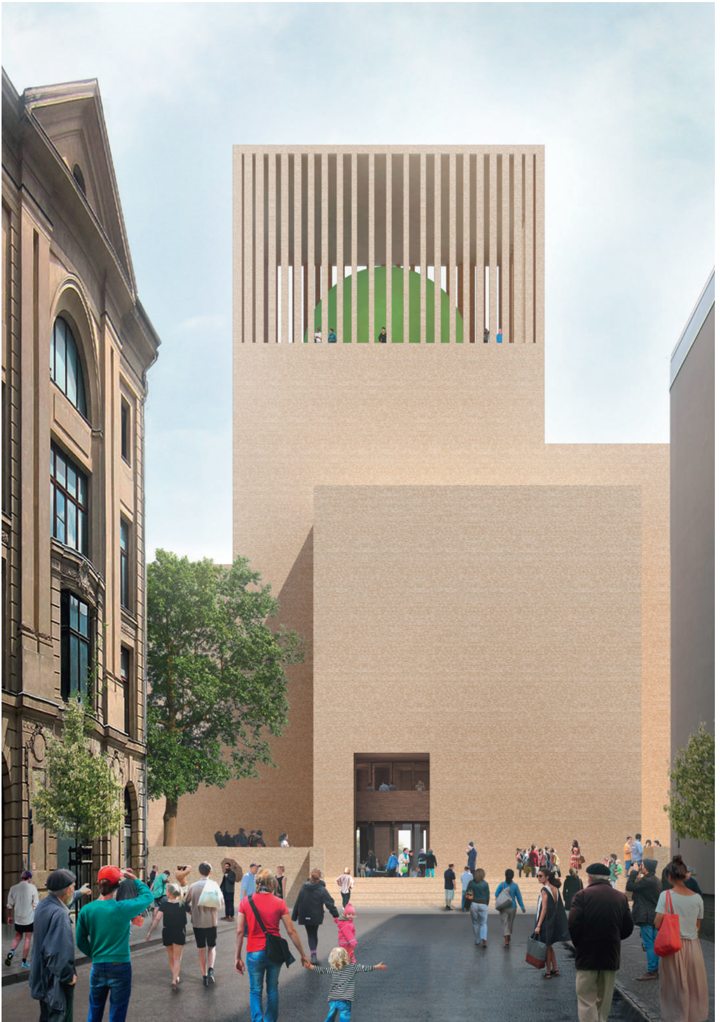
The House of One, view from Brüderstraße © KuehnMalvezzi
